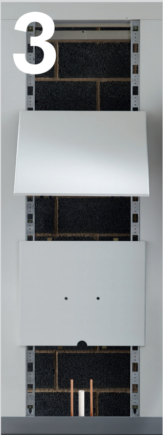
03 Drill or cut out for sanitaryware.
